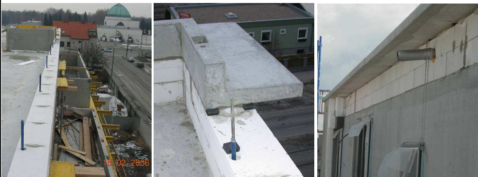
Thermic detached attic connection
